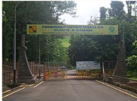
Kantor Unit PLTA Hydropower Unit Office
